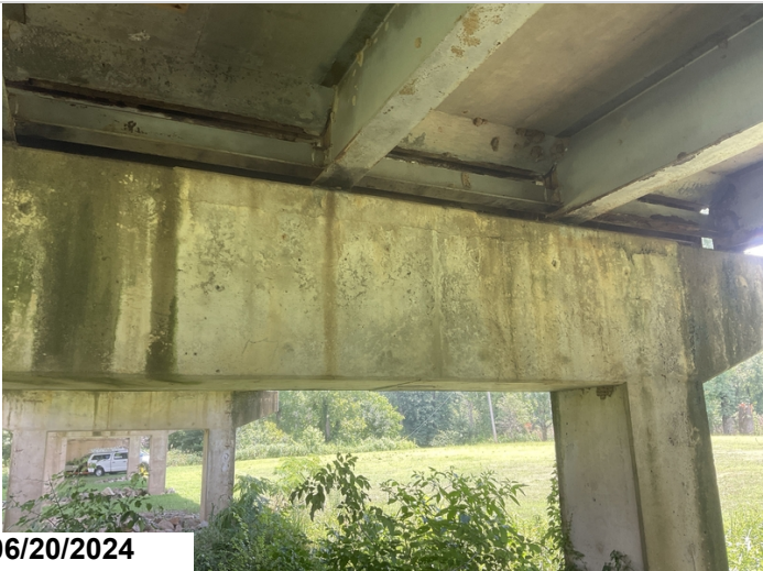
Bent # 2 has a 10' horizontal crack located approx. 6" below the top of cap.
