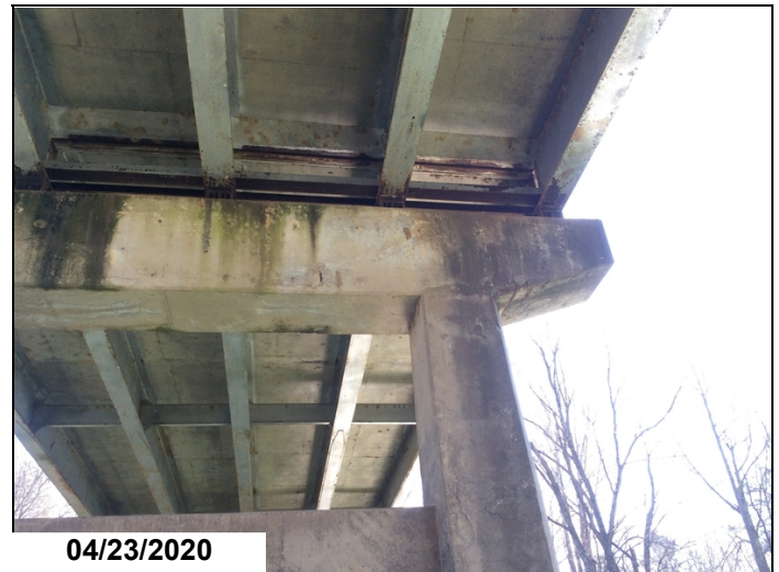
Bent # 8 spalling with exposed reinforcing steel.
