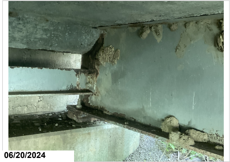
Abutment # 1, girder # 1: active corrosion and pack rust.
