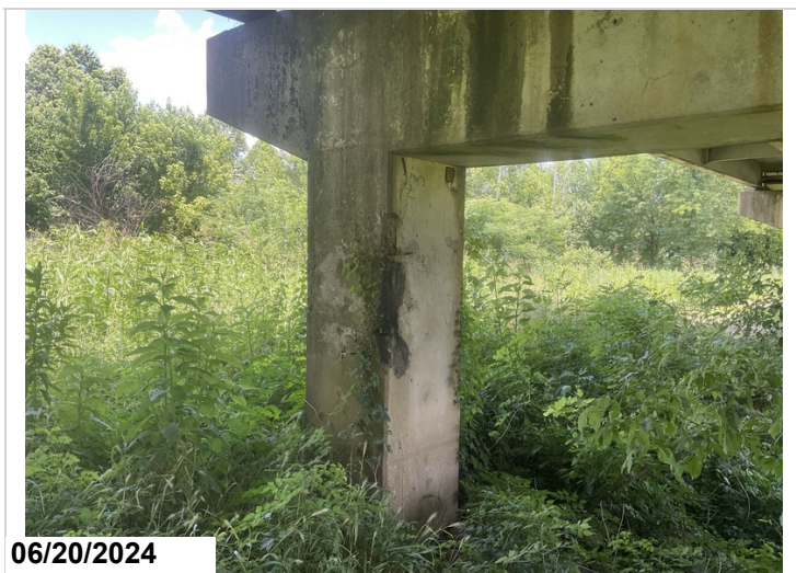
Bent # 2 has a 4' vertical spall in the Left column that has been covered with caulking as a type of repair. Concrete is delaminated adjacent to the caulked repair.
