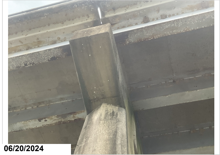
Bent # 7, left has an 18" spall with exposed reinforcing steel in the Lt underside of cap.
