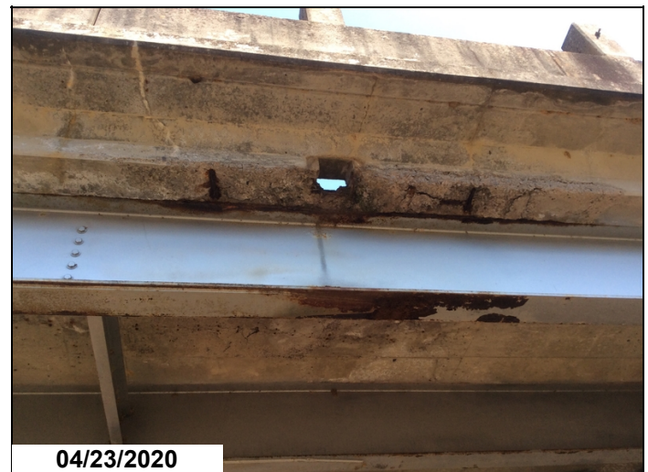
Span # 4 adjacent to beam # 5 active corrosion in the beam.
