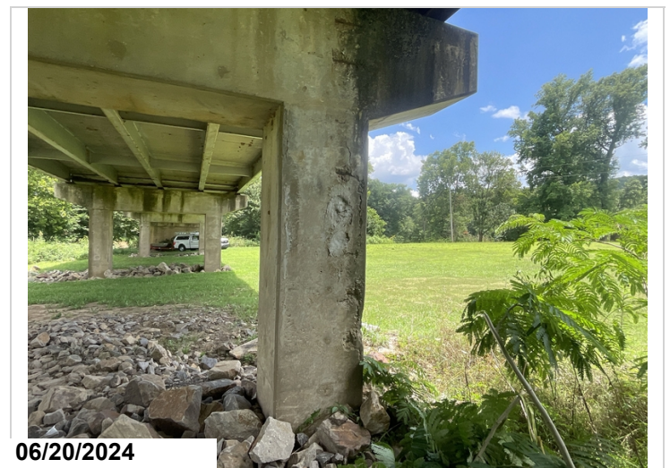
Bent # 3 has a 6' vertical delaminated area with spalls in the Right column that has been covered with caulking as a type of repair.
