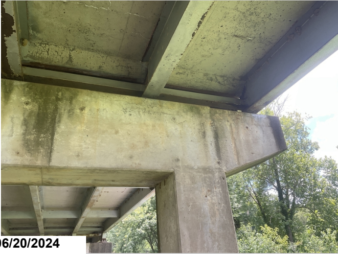
Bent # 5 has horizontal cracking approximately 6" below the top of the cap on the Span # 4 side.
