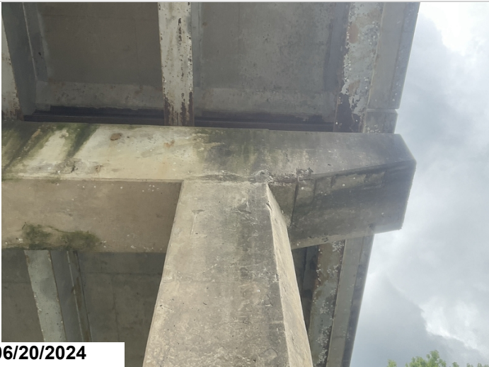
Bent # 8 has spalling with exposed reinforcing steel on the underside of the right side of the cap and on the Span # 7 face approximately 3' from Column # 2.
