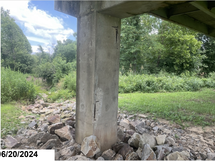
Bent # 4 has vertical cracks with spalls that have exposed reinforcing steel in both columns.
