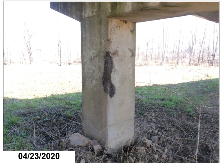
Bent # 2 Column # 1 vertical spalling filled with caulking as a type of repair.
