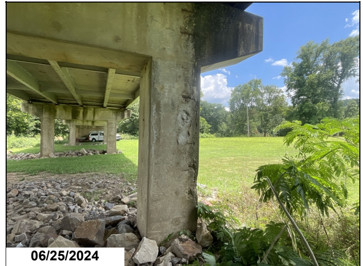
Bent # 3 has a 6' vertical delaminated area with spalls in the Right column that has been covered with caulking as a type of repair.
