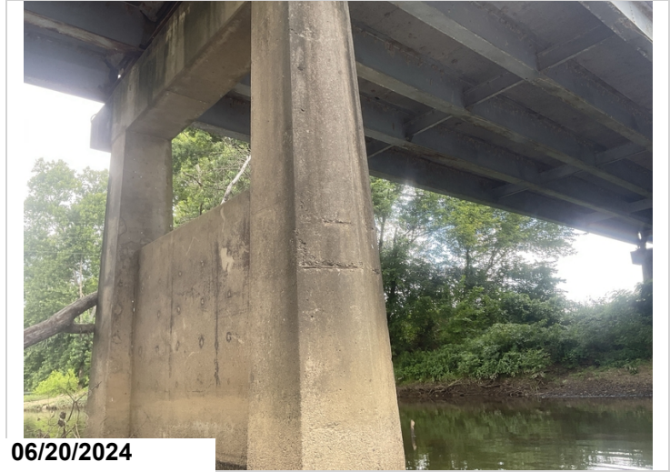
Bent # 7, Column # 1 has two 24" horizontal spalls with exposed reinforcing steel located approximately 12' below the base of cap in the Lt column.
