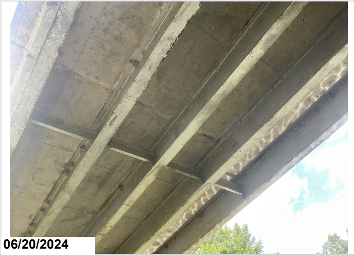
Span # 8 undersurface in bay # 3 has an 18" x 5" spall with exposed reinforcing steel located approximately 15' from bent # 8 and a 3' long delaminated area located approximately 15' from bent # 9.
