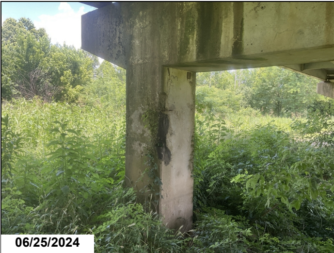
Bent # 2 has a 4' vertical spall in the Left column that has been covered with caulking as a type of repair. Concrete is delaminated adjacent to the caulked repair.
